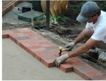
2- Laid a garden patio
